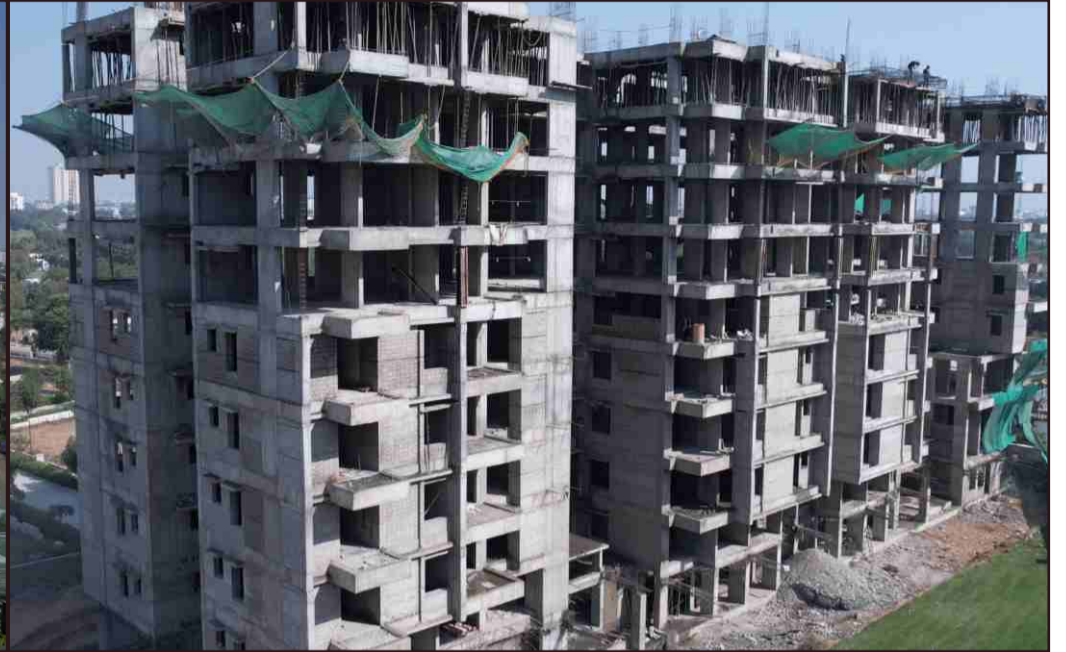
TOWER 2- ON GOING-CASTING OF NINTH FLOOR ROOF
