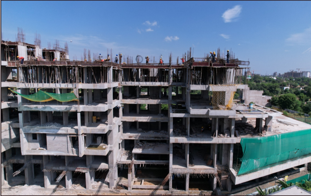
TOWER 1- CASTING OF FIFTH FLOOR ROOF
