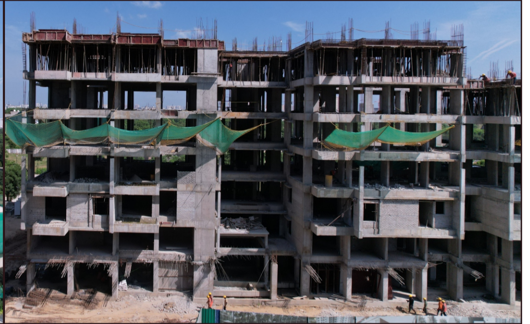
TOWER 2- CASTING OF SIXTH FLOOR ROOF
