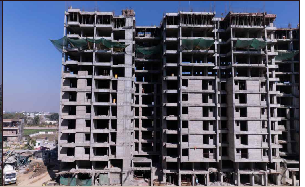
TOWER 2- ON GOING-CASTING OF TWELFTH FLOOR ROOF
